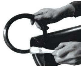
2. Lubricate gasket
