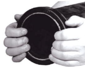
3. Gasket installation
