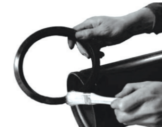
2. Lubricate gasket
