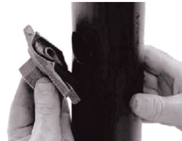
3. Gasket installation
